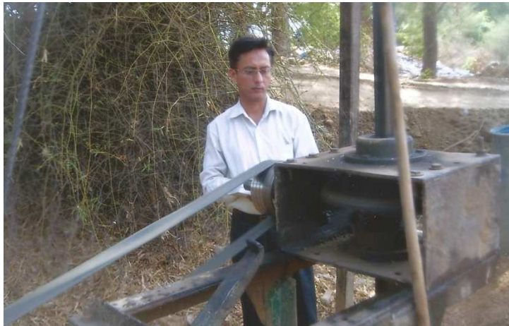
Drilling of a deep bore well in Uslapore Area of Bilaspur
